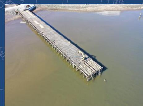
As part of the revitalization of the Borough of Carteret and the shorelines, the Mayor of Carteret requested to inspect, evaluate, and provide recommendations for repair or replacement of an existing and deteriorated 540' long timber pile bent pier within the Arthur Kill. The pier is estimated to be built in the 1920's and was originally used as a loading dock with crane rails for large vessels unloading shipments to the industrial areas along the Arthur Kill.
